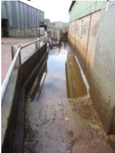
Photo1: A built in concrete footbath is more comfortable for the cows to walk through and less disruptive to cow flow.
